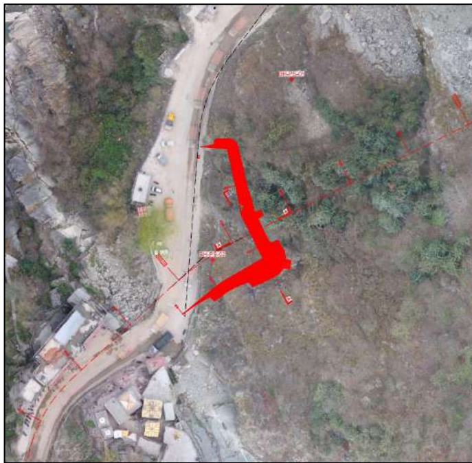
Figure 34 - South Portal Area
