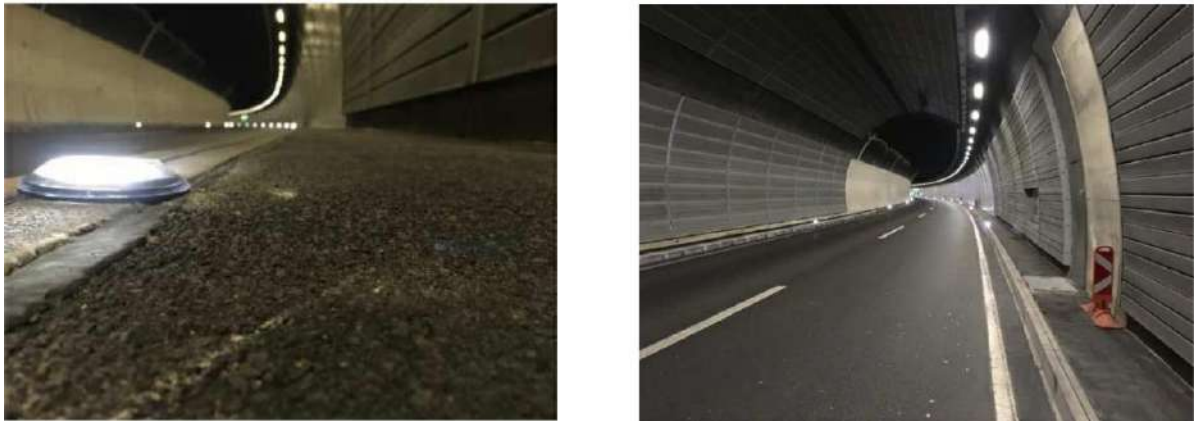
Picture 4: Example of LED optical guide
