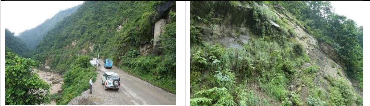
Fig. 4 : Rockfall events recorded during time along Siddababa highway (Gyawali et al. 2015)
