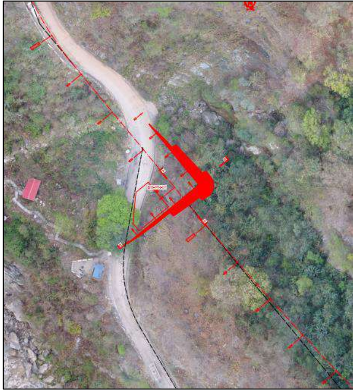
Figure 33 - North Portal Area
